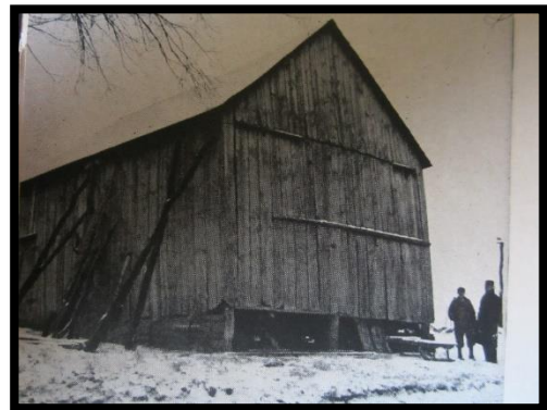
"The Leaning Barn"
